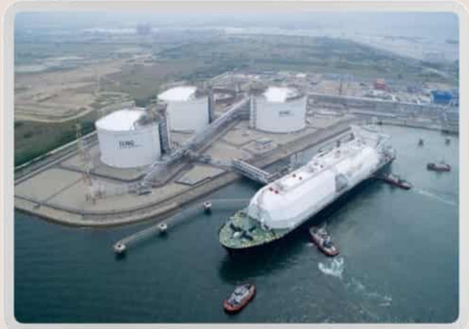
The Singapore LNG Terminal (Source: STE What's Next)
